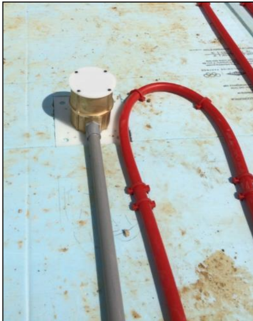
Sensor socket before concrete
