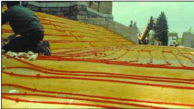
Spray-foam insulation on old stone steps (church)
